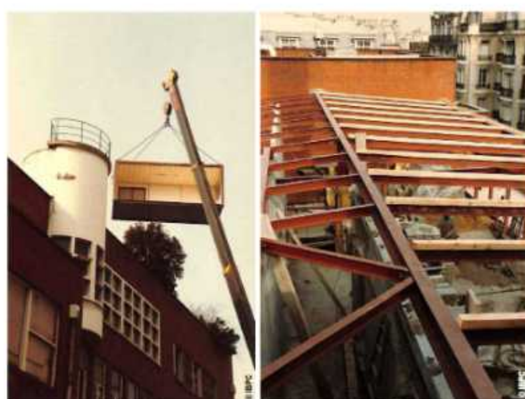
INSTALLATION DE LA CAFÉTÉRIA TEMPORAIRE INSTALLATION OF TEMPORARY CAFETERIA
