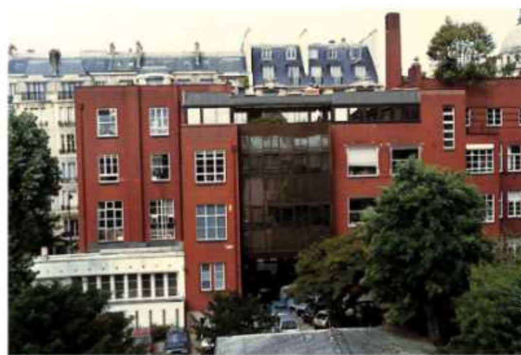
L'IBPC RENOVÉ FAÇADE SUD THE IBPC RENOVATED SOUTHERN FACING SIDE
